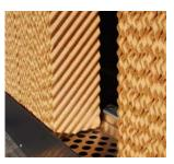
When evaporative pre-cooling is required, a highly absorbent media is wet using city water. The honeycomb design provides a large wetted surface that is exposed to the entering air to provide maximum adiabatic effect to lower the incoming air temperature. 6" thick media is used to provide the required performance. Excess water
